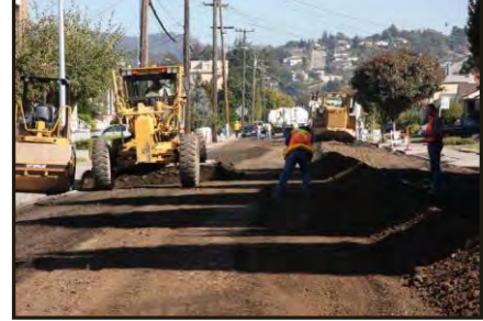
3. RESHAPE FOR NEW HMA OVERLAY
