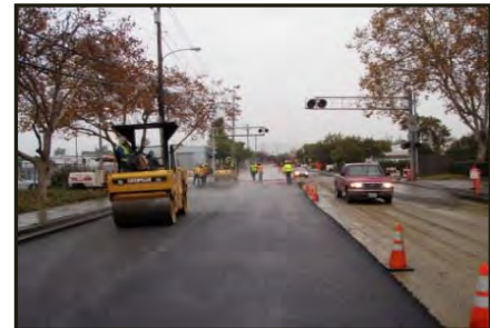
9. OVERLAY NEW HMA
