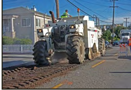
2. PULVERIZE DETERIORATED PAVEMENT
