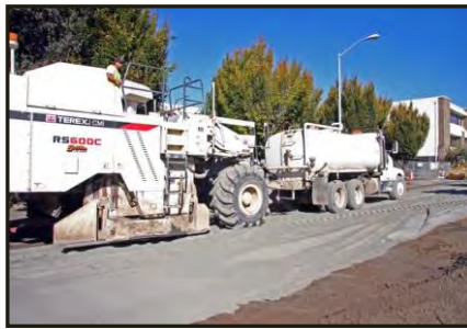
5. MIX – HYDRATE CEMENT & RECYCLED BASE
